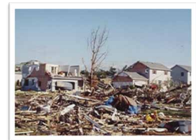
Figure 4.5 Damage in the Capital District from May 31, 1998
